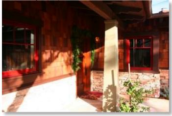
This is a picture from my front porch which has the same columns as the rear. The columns are square and taper from the bottom to the top. Measured along one side of the column, the top is 10" and the bottom is 15". The columns are 8 feet tall.
