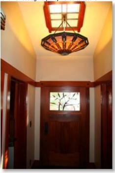
This is actually a custom door of my own general design with final design by the woodworker, Joe Madden. It is solid mahogany, 2.25" thick, 42" wide, and weighs 150 lbs. As you can see on the web site, I made the stained glass about a year after the door was in. I had the door made with a removable frame that slides into place and is held in by 3 screws at the bottom. This way I can swap out the glass at any time. The manufacturer was Joe Madden of Madden Millworks in San Pedro, CA.
